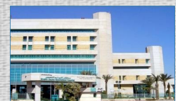
ZAYED HOSPITAL ( A.H.U / CU )
